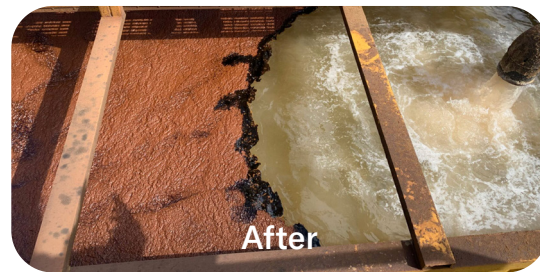
Noticeable increase in floc size/tightness plus improved water clarity and separation from oil
