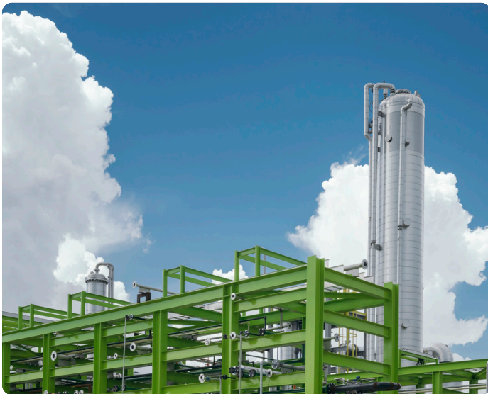
Solugen's first-of-its-kind Bioforge™ plant in Houston, TX.
